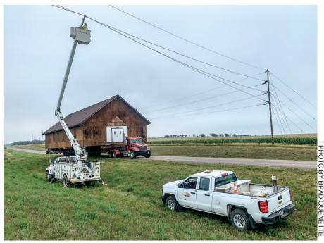
In August, some linemen lifted transmission lines in the Beulah area to accommodate the move of an old church. Switching of power feeds was required for this project. Assisting in requests like this, and making sure the move was safe and efficient, is just one way Roughrider shows its commitment to community.
