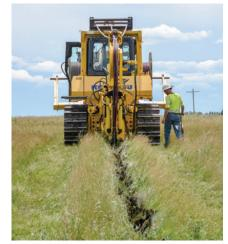
Foreman **Doug Roethlisberger** walks behind the plow train to make sure the cable is placed as planned. The plow train rumbles along at a steady pace, unless it hits rock and needs to slow down to slice through the barrier.
