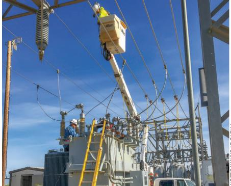
Maintenance plays an important role in system reliability. In June, Electro Test did transformer bushing maintenance with our line crews. Roughrider Lineman Cody Hintz is in the bucket. This photo was taken at our Schefield Substation.
