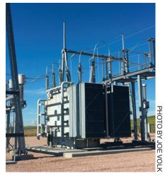
"Dressed" with accessories and oil at the Rhame Substation prior to the move, the transformer weighs 306,900 pounds.
