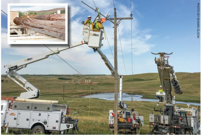
Roughrider Electric Cooperative linemen prepare to change out a damaged pole, working the lines "hot." We keep the lines energized, when possible, so our members have uninterrupted electric service. Replacing the compromised pole prevented a potentially lengthy outage. Pictured here are Linemen Tyler Phelps (left) and Dion Gefre, who are applying cover-up and grounding in the buckets, and Mike Steier, who is operating the digger.
