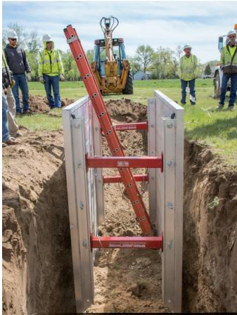
A trench box, also called a trench shield or trench sheet, is a steel or aluminum structure that is used to protect utility workers while performing their duties within a trench. Customarily constructed with sidewalls of varying thickness held apart by steel or aluminum spreaders, the box can withstand a collapse without buckling.
