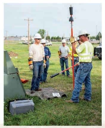
Kyle Irwin (far left), journeyman lineman for Roughrider Electric Cooperative, watches an underground splice repair mid-span, in which the linemen discussed insulation and isolation, and grounding methods for that particular work.
