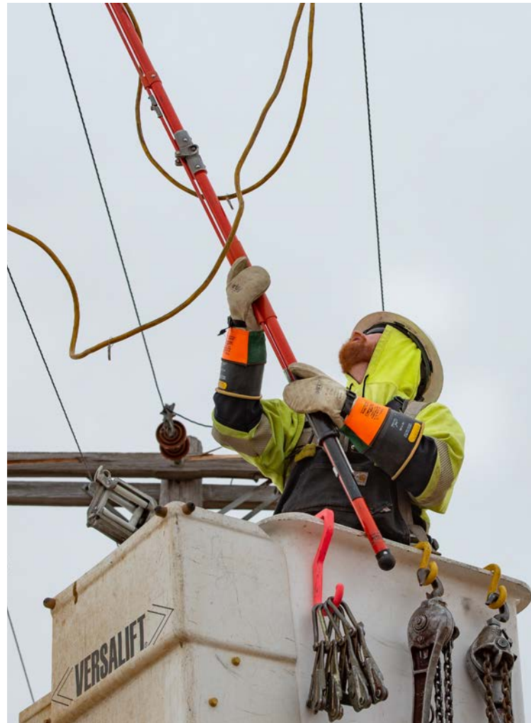
Lineman Tanner Goetz adds protective grounds to protect line crews from possible dangerous voltage back feed on the line.
